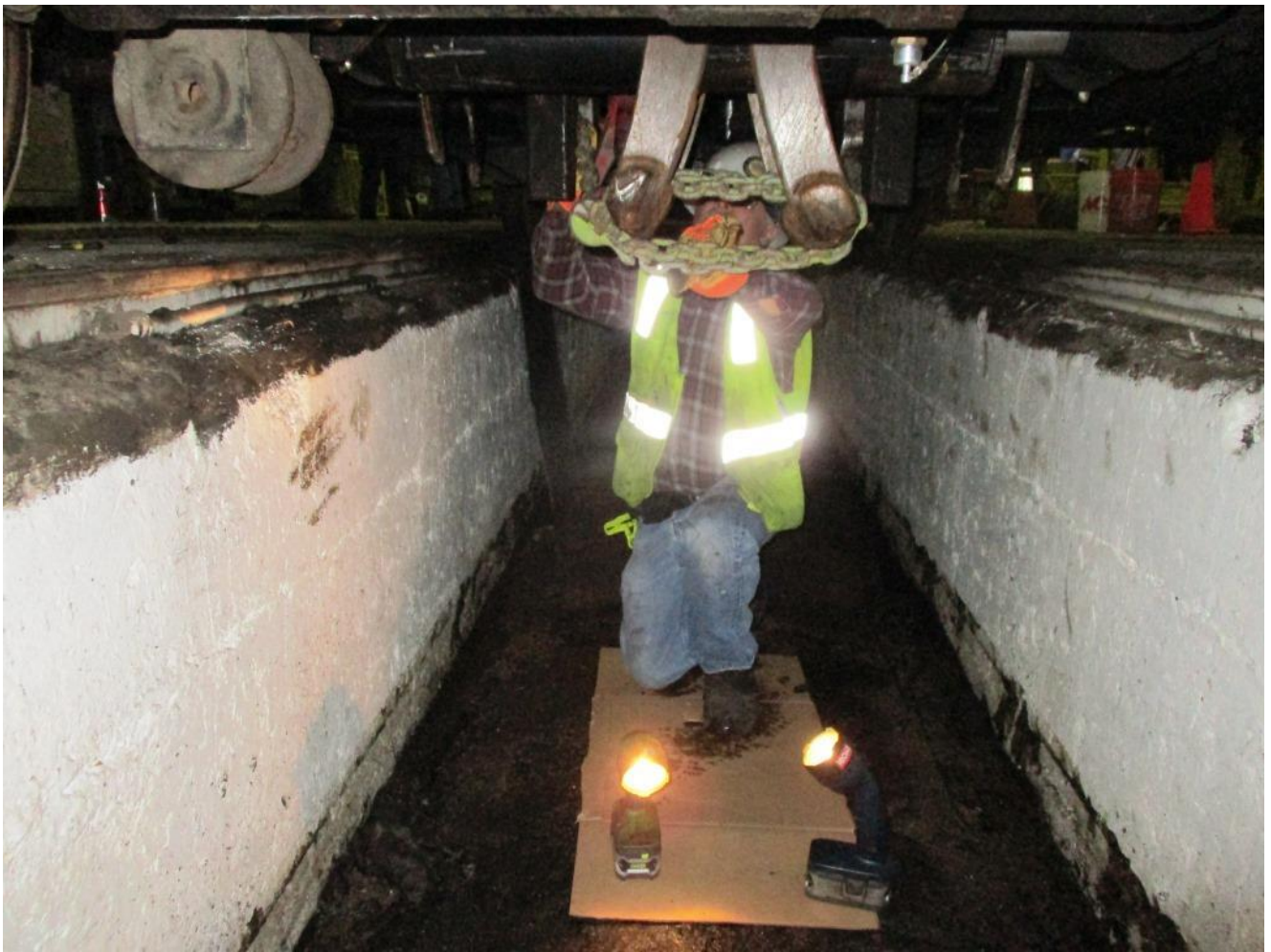
Under the tie-shear, Mike H. works to remove the kickers' cylinder
