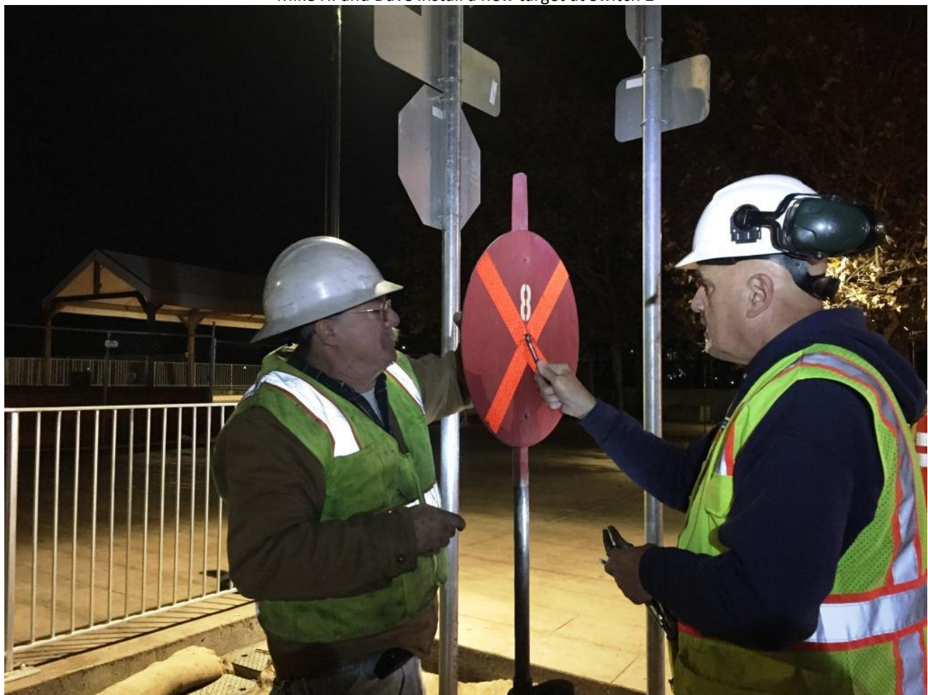
Mike H. and Dave remove the old target at Switch 8
