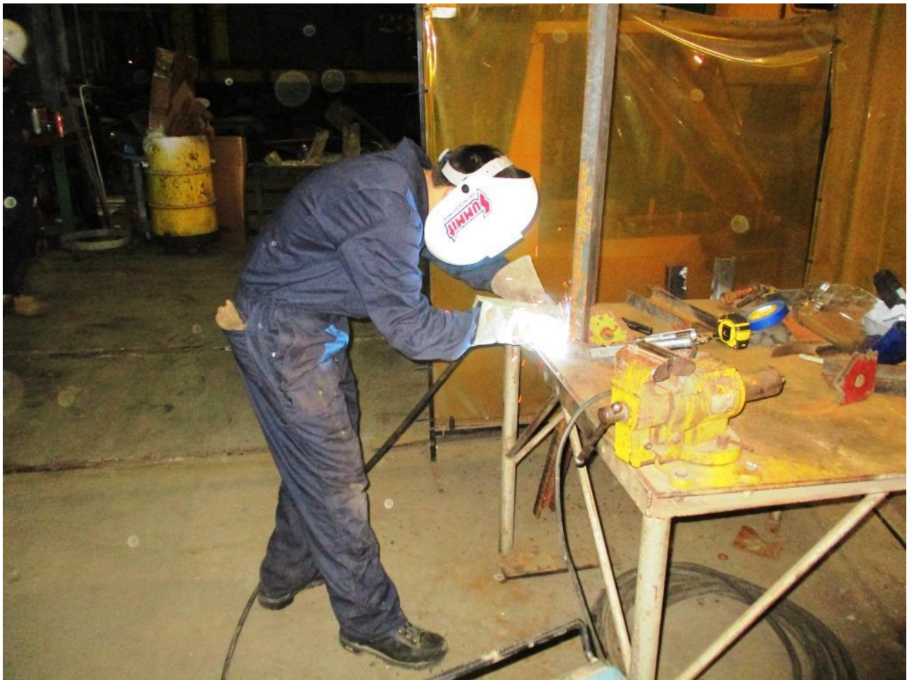
Kyle welds together the new mounting bracket for the Nolan track-cart to be placed on the air-compressor
