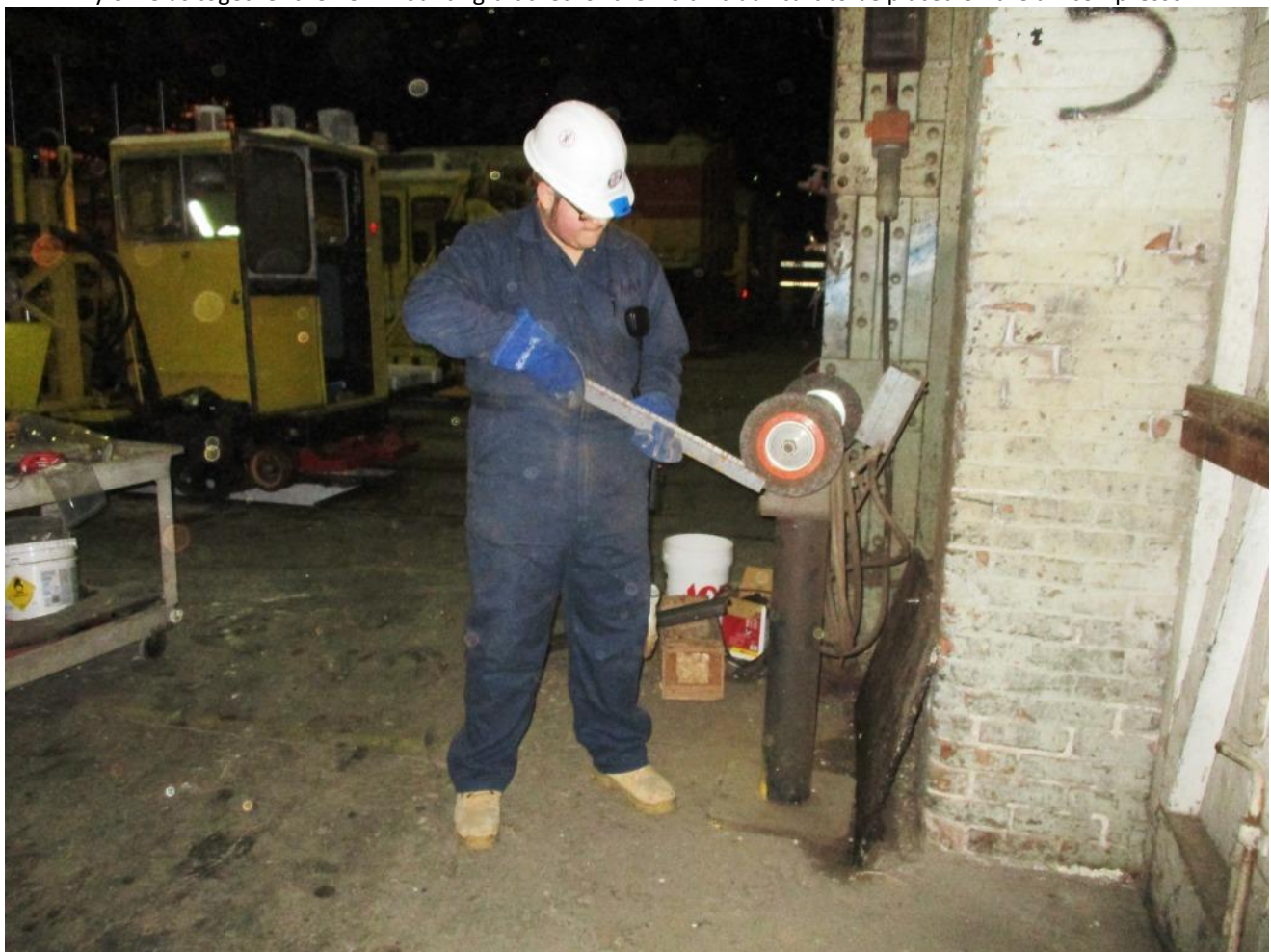
Chris H. uses the wire-brush on the area to be welded
