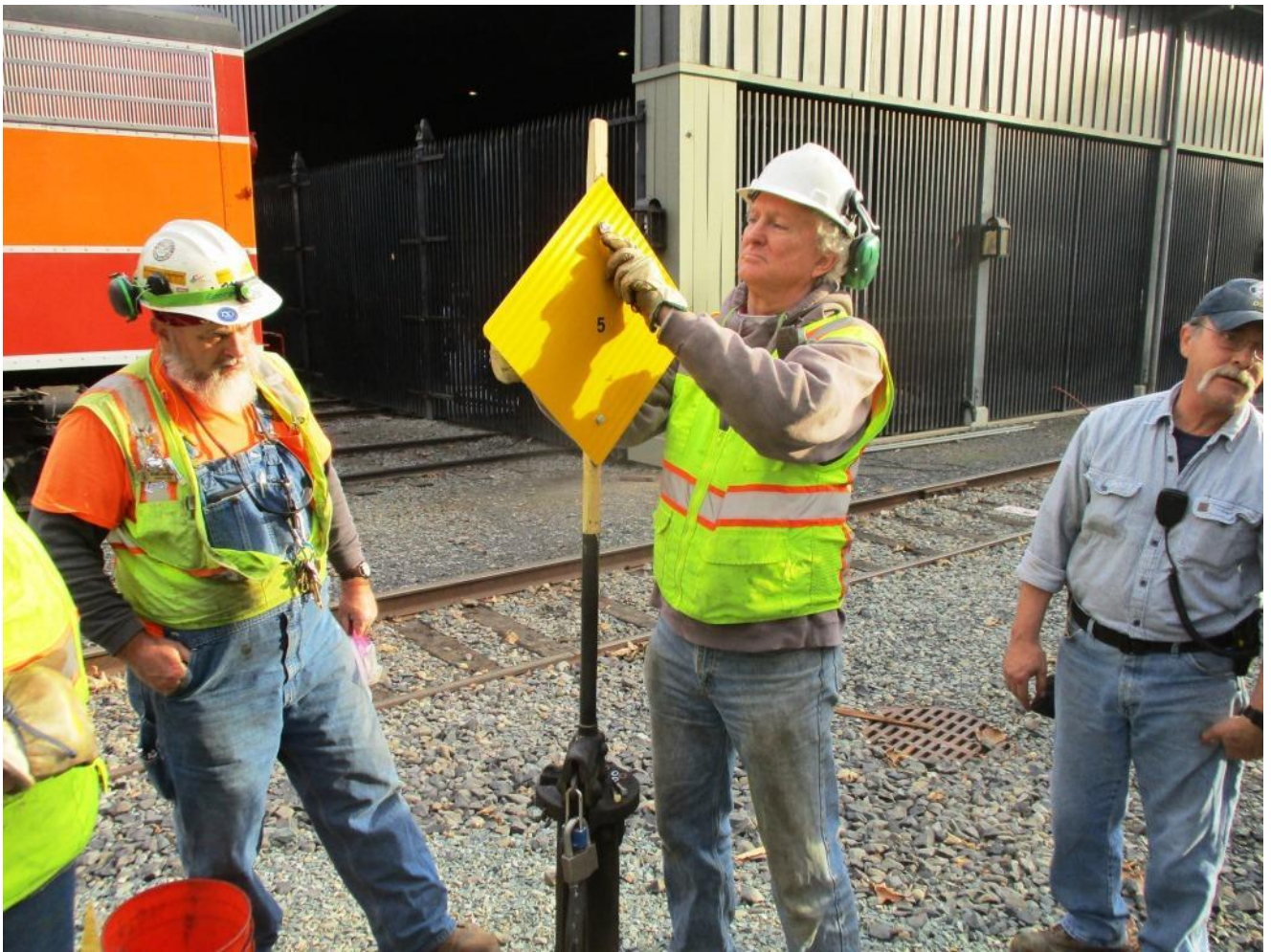
Steve installs the new target at Switch 5
