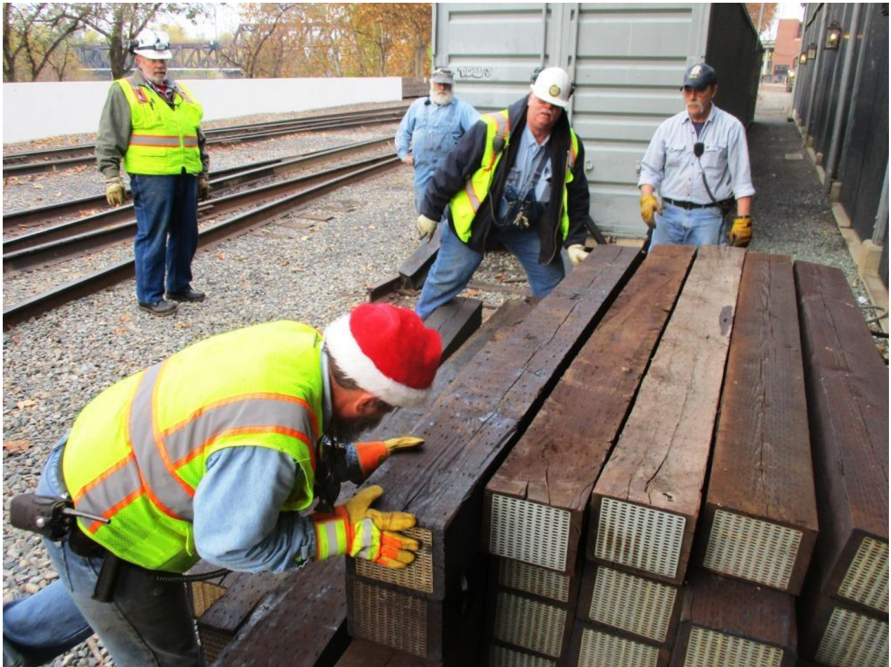
Joe, Chris, and Jeremy get the pile of heavy, hard-wood ties orderly for GM2 to pick up
