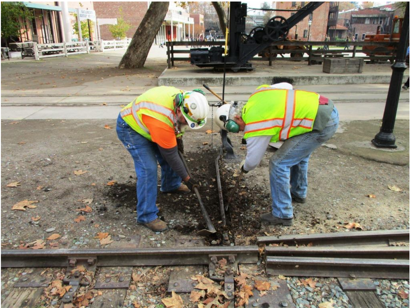
While all the excitement is going on with the 125, Mike F. and Steve clear debris away from the control rod of the Stub Switch
