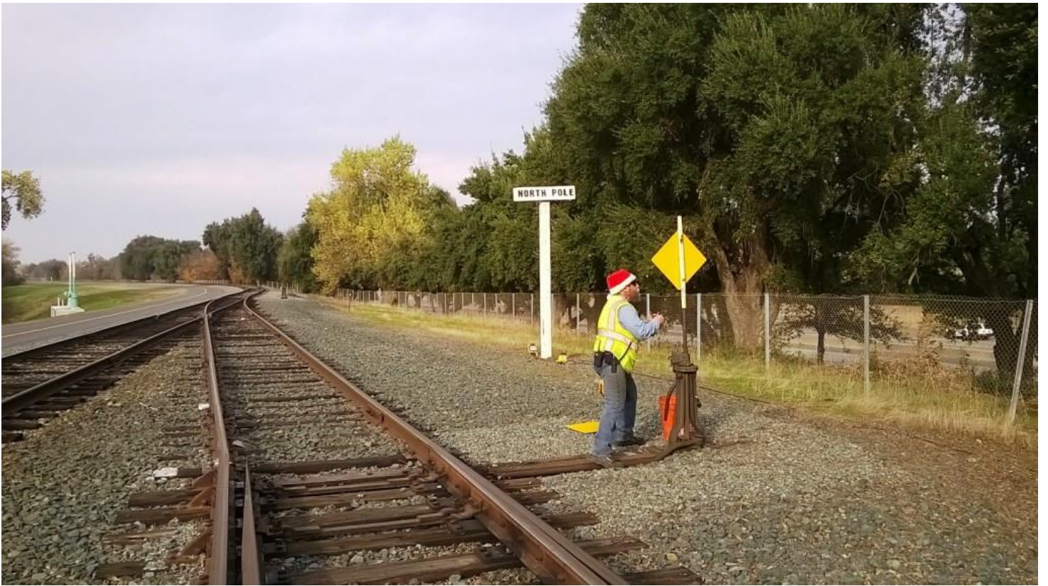
At Baths, Joe replaces the old, faded, ugly target on Switch 18 with a fresh, new, highly reflective target
