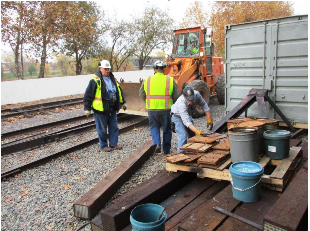
Chris, Art, and Jeremy load tie-plates into the bucket of the front-end loader
